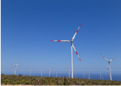
Los Cururos | 109MW Acquired in 2019
