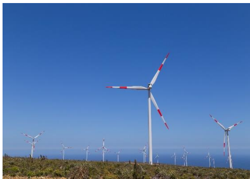
Los Cururos | 109MW Acquired in 2019
