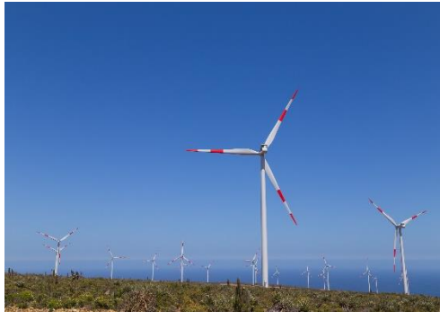
Los Cururos | 109MW Acquired in 2019
