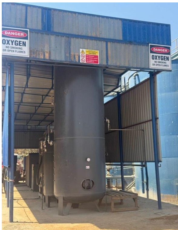
Figure 2: Additional capital plant expansion works
