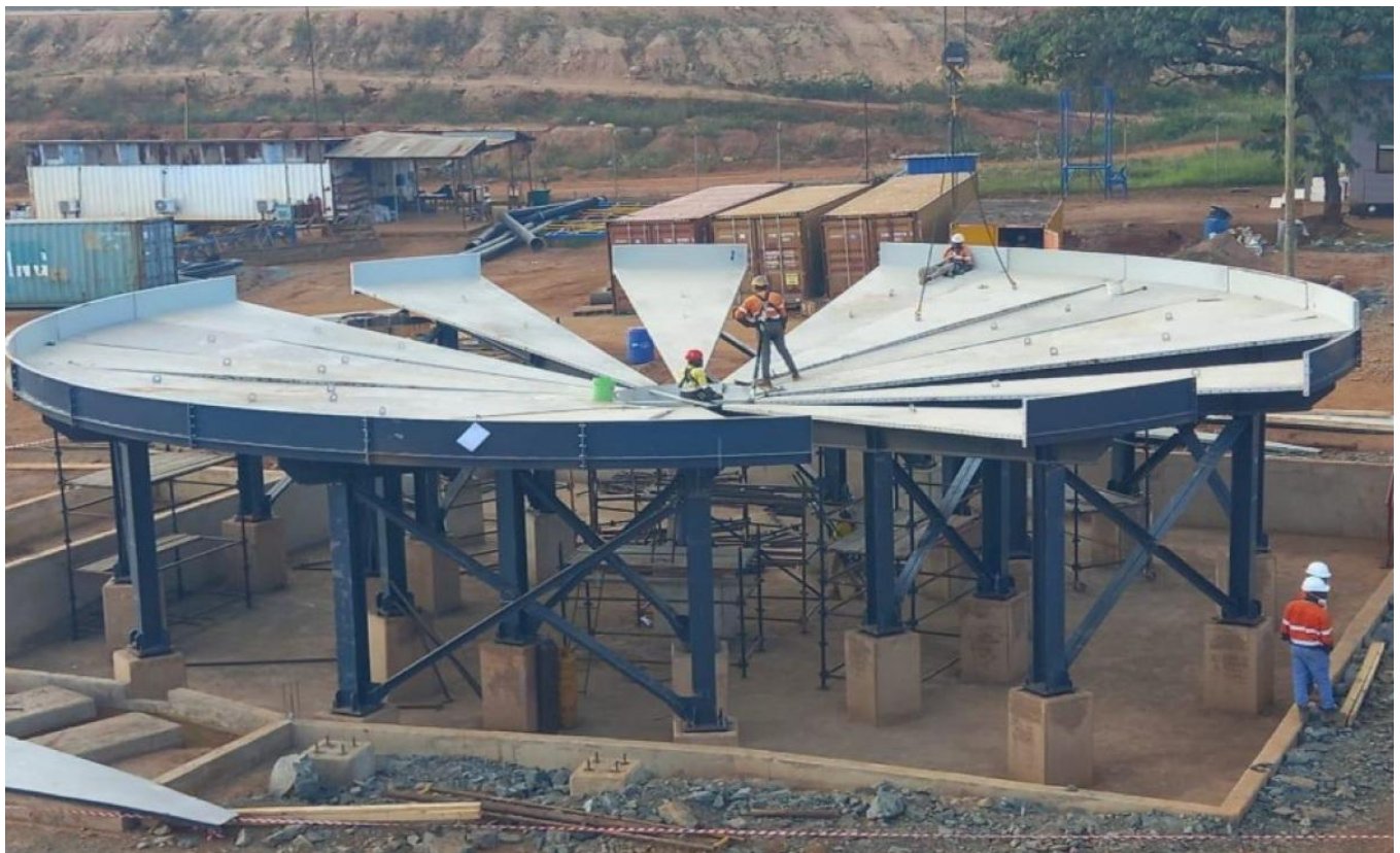
Figure 2: Additional capital plant expansion works
