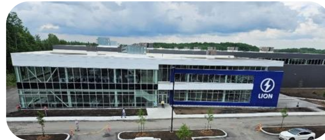
BATTERY PLANT IN MIRABEL, QC
