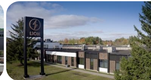
MANUFACTURING FACILITY IN ST-JEROME (MONTREAL), QC
