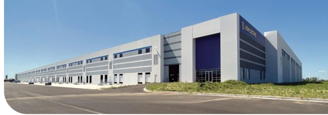
MANUFACTURING FACILITY IN JOLIET, IL
