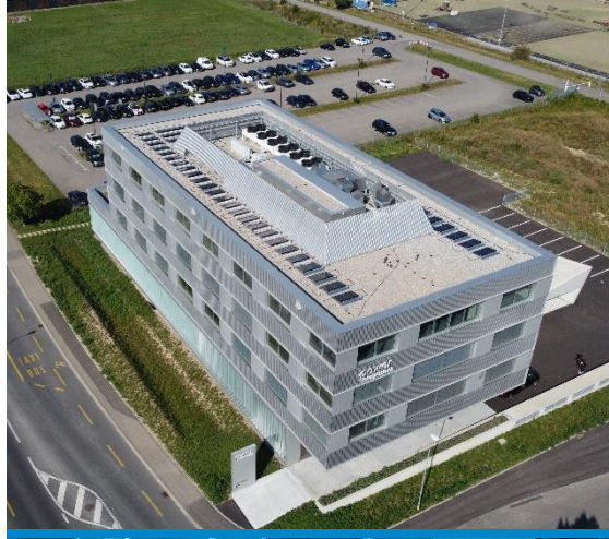
25 kW at New Switzerland Facility
