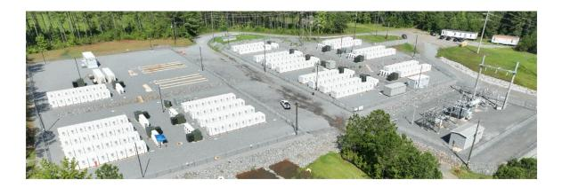
Georgia Power worked with industry leader Wärtsilä to provide the engineering, procurement and construction services for the Mossy Branch facility. The project utilizes the GEMS Digital Energy Platform, Wärtsilä's energy management system, to manage the facility and provide secure operations, and is built with Wärtsilä's Quantum, a fully integrated, modular, and compact energy storage system.
